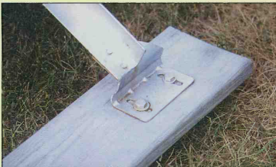
Here's a close-up of the bed frame footing where it's bolted to the weatherproof wood.
