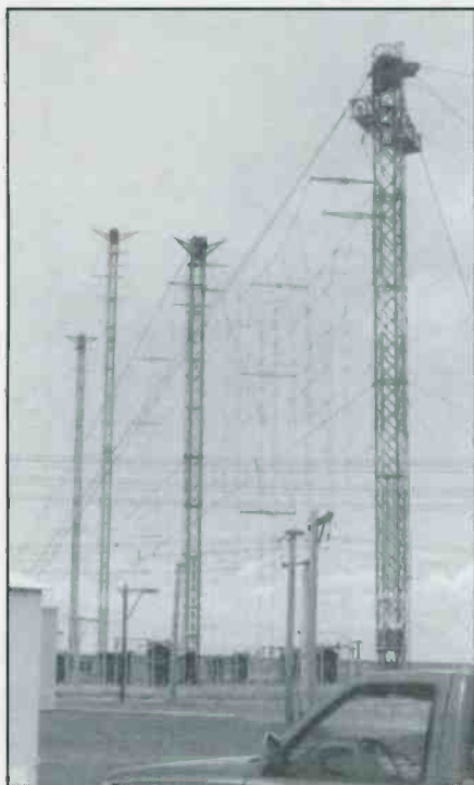
Here's a part of the transmitting facility at RCI, Sackville, New Brunswick.
