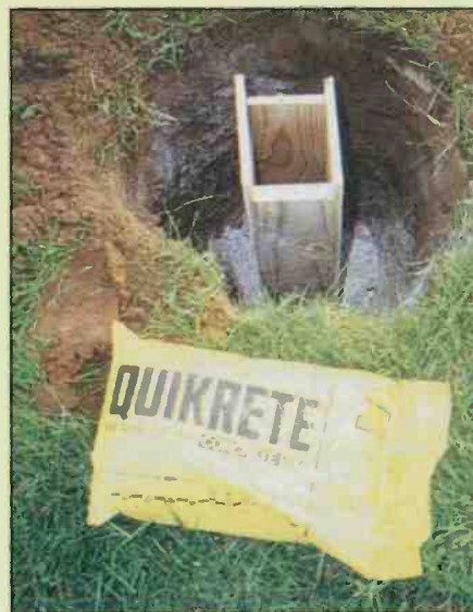
If you decide to mount a panel in the ground, be sure the buried cement wall is large enough to withstand the stress of your pole-mounted panel.
