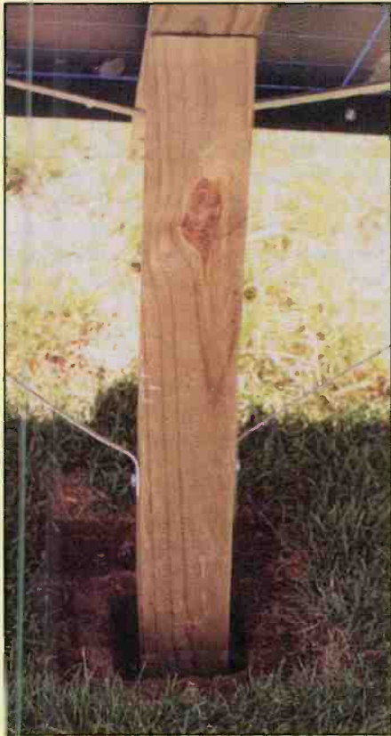
The two panels mounted on the fencepost are inserted into the hole.
